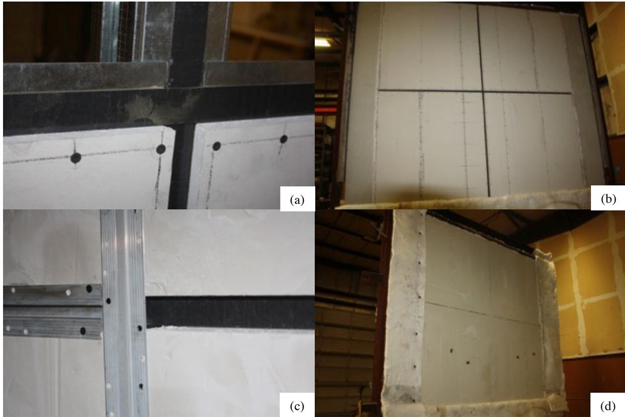
Figure 1. Construction photographs showing (a) center FSB joint with single layer of GWB, (b) wall before compound, (c) installation of DRM trim, and (d) completed assembly.
