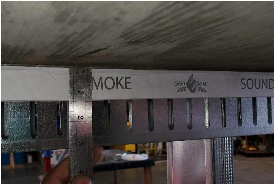
Figure 2: 1-1/4 inch Safti-Seal Smoke-n-Sound Gasket installed on the top track.
