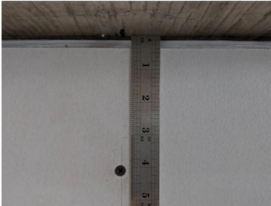
Figure 4: The assembly was constructed with a 3/8 inch Head of Wall joint.
