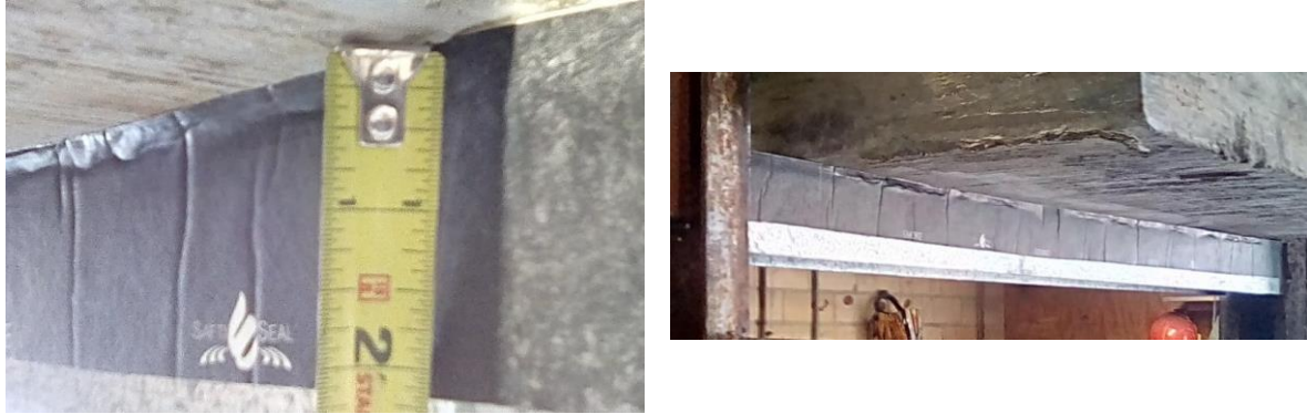
Figure 2: On the left the SSG is shown to be 2-1/4 inches wide. On the right the SSG is shown adhered to the ceiling runner/top track.
